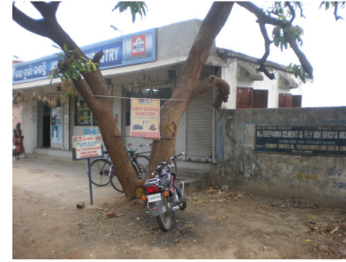
Use of land for partly commercial purpose though leased for industrial purpose (Seepona Cement and solid Brick), Paramanandapur, Kalahandi District
