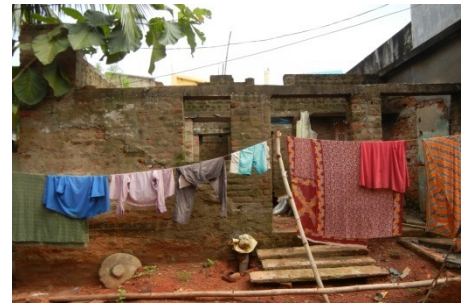
Delay in completion of dwelling units at Bharatpur slum noticed on 12 Sept. 2011
