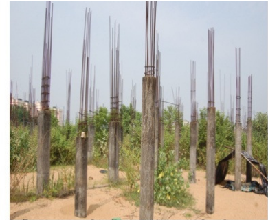
Interrupted construction work of Kalamandal building on a disputed land at Bhubaneswar
